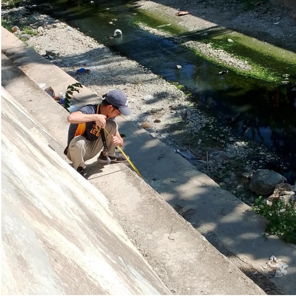
Fig 2.3 Measurement of old riprap in this area is 270 - 300 cm
